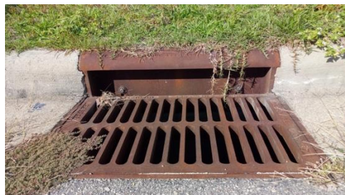
Photo of a storm drain
