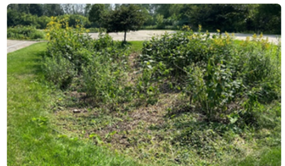
After photo: once woody vegetation and invasives were identified and removed, the basin needed to be replanted with native plant plugs to fill in bare areas.
