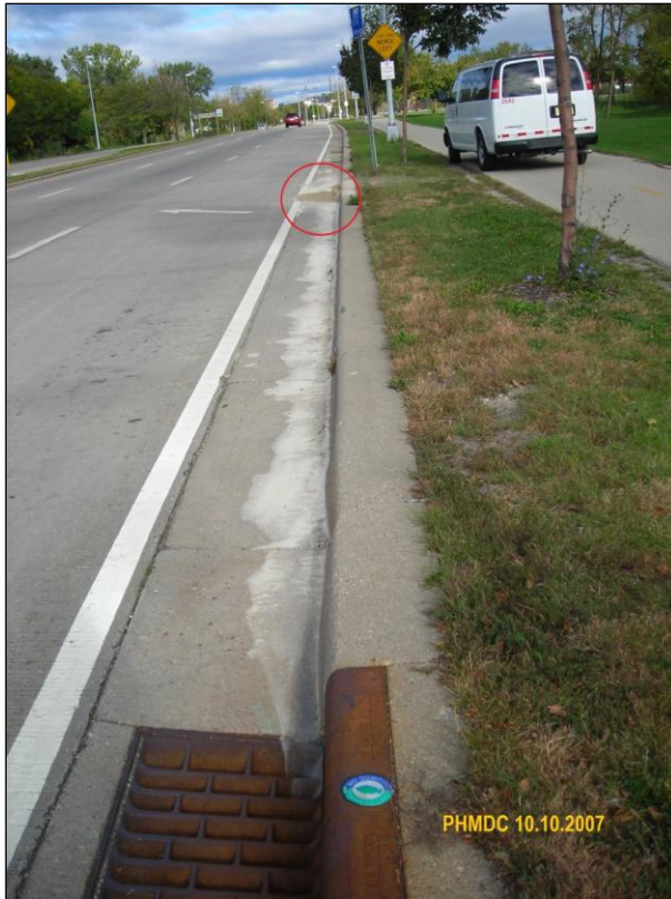
Photo 2: concrete-truck chute washout. Chute was washed in the circled area. Note the pile of coarse material. Contaminated wastewater flowed to storm sewer.
