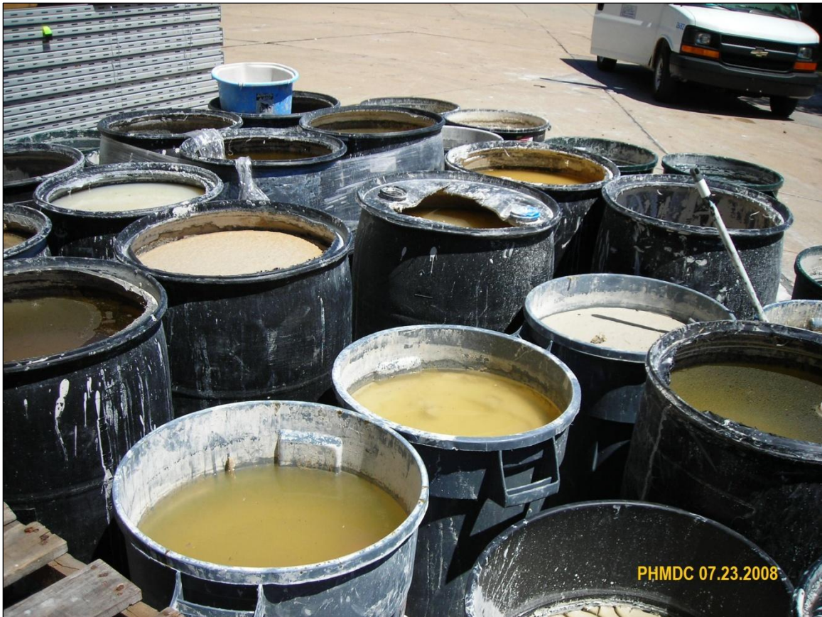
Photo 16: unsecured concrete slurry.
