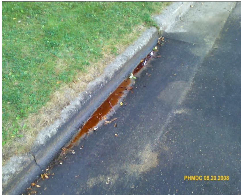
Photo 12: pooled transmission fluid in the gutter.
