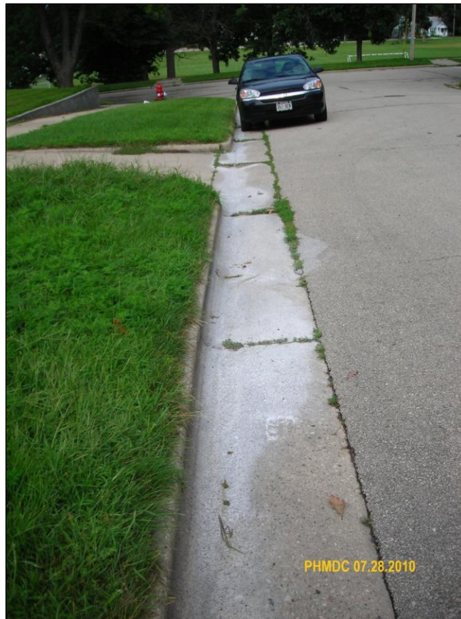
Photo 7: telltale staining from paint tool washing.
