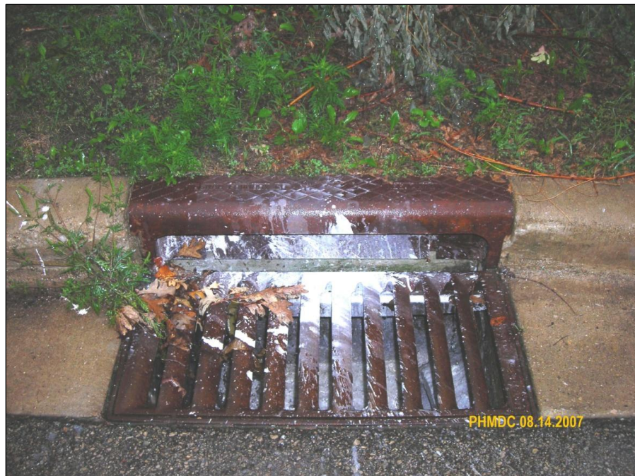
Photo 8: dumping of leftover paint from a roller tray.
